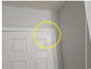
9.5 Item 7(Picture) Front Right Bedroom
