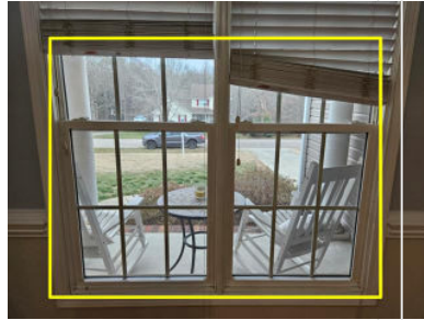
2.2 Item 2(Picture) Dining Room
