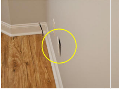
6.4 Item 4(Picture) Front Right Bedroom
