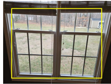
2.2 Item 5(Picture) Master Bedroom
