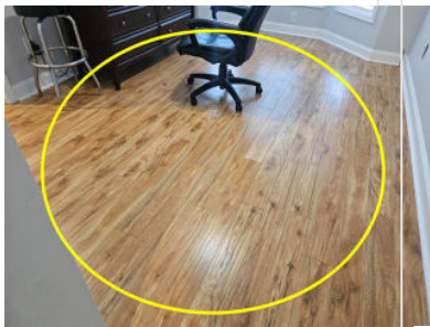
4.1 Item 6(Picture) Front Right Bedroom
