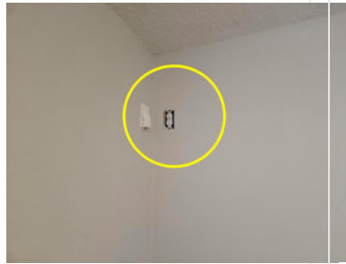
6.4 Item 7(Picture) Rear Right Bedroom
