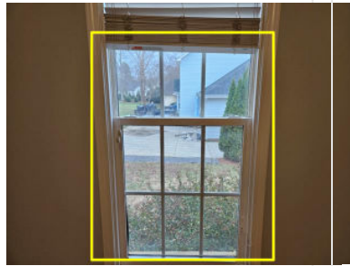
2.2 Item 4(Picture) Rear Right Bedroom
