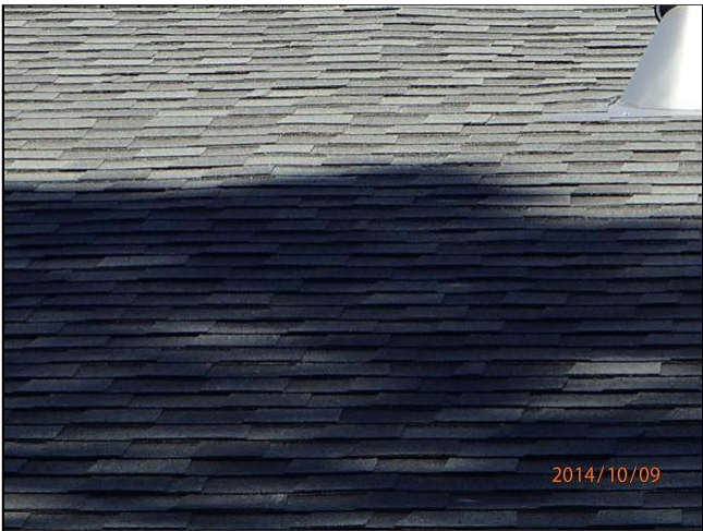
Complimentary Roof View
