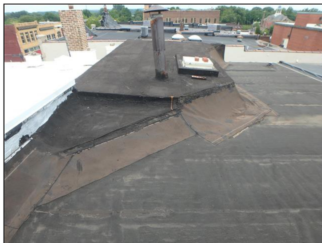
Complimentary Roof View
