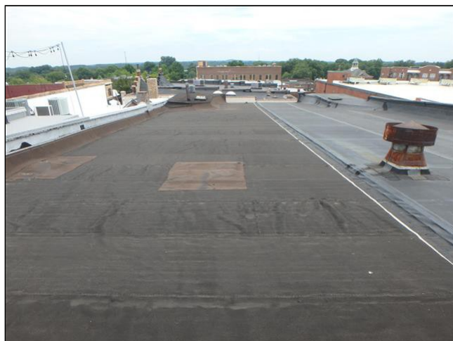
Complimentary Roof View
