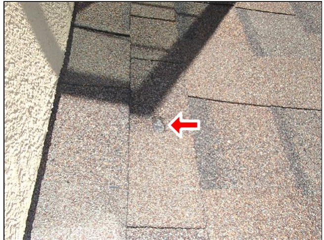
Ridge Cap Shingles Damaged
