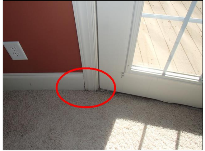
Rear Entry Door Master Bedroom
