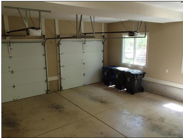
1st level garage views
