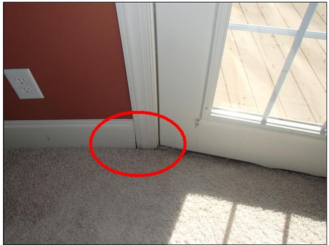
Rear Entry Door Master Bedroom
