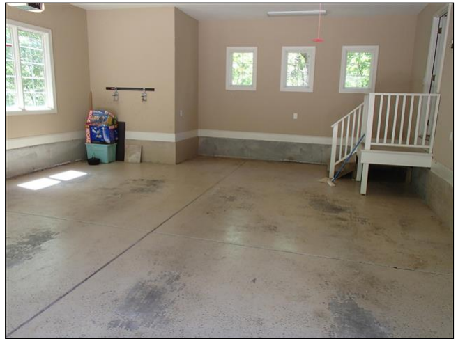
1st level garage views
