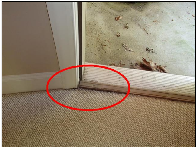
Rear Entry Door (Office)
